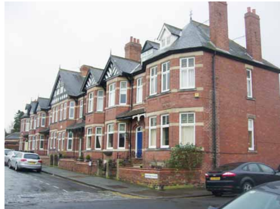
A variety of bays (single and double) integrate to create high and low half timbered gables, interspersed with individual dormer windows. The resultant building group is complex and over fussy, yet offers a good example of exuberant Darlington Edwardiana.
