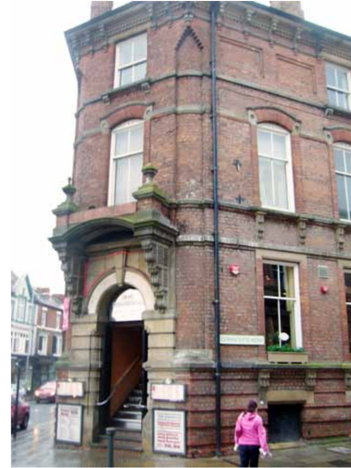
Corner turners - Entry doors and fenestration overlooking the junction are strengthened by panelled brickwork and decorative stone 'band courses'
