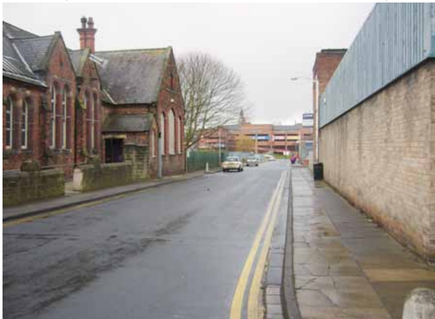
Brunswick Street links back to the Town Centre and may provide important pedestrian links to Central Park in the future. Victorian School buildings, currently used as a music centre off Brunswick St create valuable key buildings within a resurgent streetscape.
