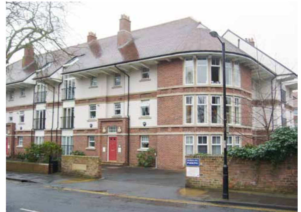
'Historically referenced' detailing - Steep roofs, chimneys and deep eaves; with articulated soffits. Render and brickwork with art-stone bound courses. Windows with 'Edwardian' astragals and glazing bars. Articulated entrance doors
