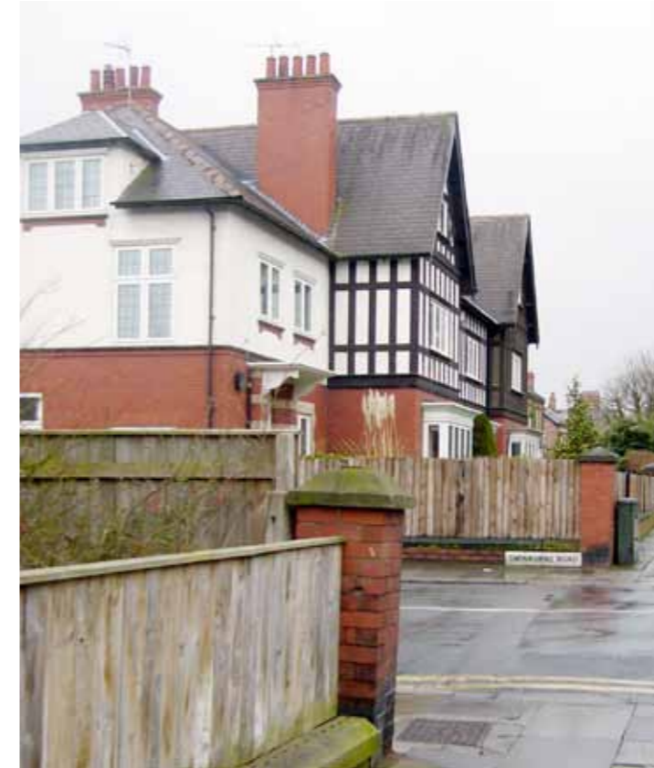
Accrington red brickwork contrasts strongly with black and white half timbering. Entrance porches are first-topped, as are the bay window roofs
