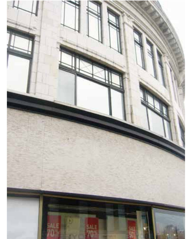
Corner turners - Darlington has a number of precedents where the curved building facades carry the eye around the corner. In this instance the buff coloured faience work is supplemented with buff mosaic
