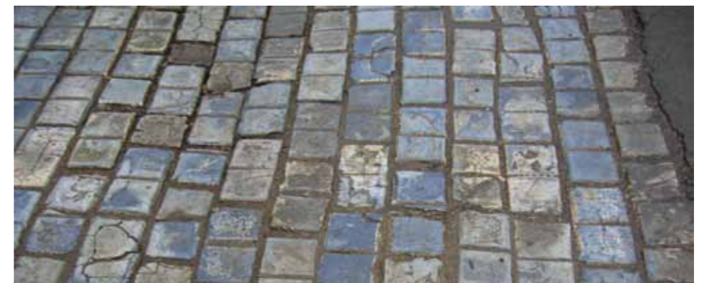
Scorria blocks - Scorria blocks are a by-product of the Teeside iron industry. These hard wearing ceramic bricks offer subtle blue and green hues and are often encountered as a traditional edging for roads and pathways
