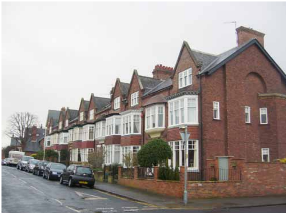
Typical Darlington Edwardian terraces. Gabled dormers create an articulated roofscape. Alternating bays and ariel windows provide modelling to the facade
