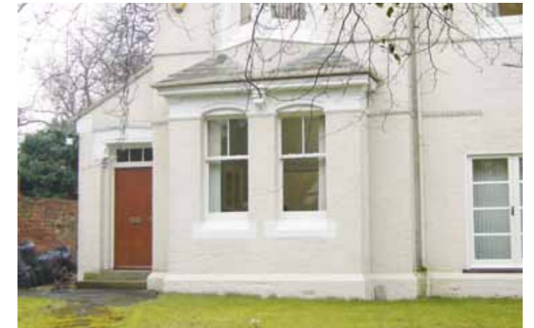
Bay windows with oriels above create 'corner turner' features
